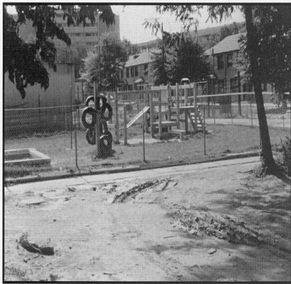
Figure 11.21b Fencing as an Interim Control for Bare Soil Hazards.
