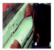
Paint affected by the mildew is deteriorated paint and must be repaired when an adhesion test determines that any layer is not securely bonded. To conduct an adhesion test, firmly press a 2" x 2" piece of masking tape to the suspect paint and rub the tape to adhere firmly. Lift up on one corner of the tape and remove the tape. If paint is evident on the tape, the paint is separating from the substrate or from underlying paint, and is not securely bonded.
