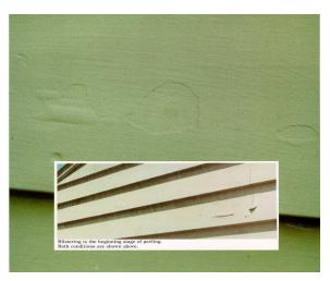
Blistering paint is deteriorated paint and must be repaired.
