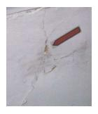
Paint that is not securely bonded is deteriorated paint and must be repaired. To conduct an adhesion test, firmly press a 2" x 2" piece of masking tape to the suspect paint and rub the tape to adhere firmly. Lift up on one corner of the tape and remove the tape. If paint is evident on the tape, the paint is separating from the substrate or from underlying paint, and is not securely bonded.
