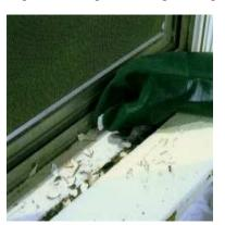
e. Painted Friction or Impact Surface. The friction and impact surfaces are evidenced by worn or chipped paint. The friction and impact of these surfaces can also result in dust–lead, which is not detected in a visual inspection.
