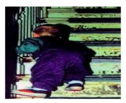
Worn paint is often due to improperly hung doors, sticky window sashes, sticky drawers, etc. A source of dust–lead are windows that do not operate smoothly and doors that bind or otherwise contact the frame. To test for friction surfaces open and close painted doors, drawers and windows. Visually inspect doors, windows, trim, floors and stairs for evidence that the paint is worn or chipped.
