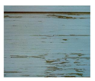
Checking paint is deteriorated paint and must be repaired when an adhesion test determines that any layer is not securely bonded. To conduct an adhesion test, firmly press a 2" x 2" piece of masking tape to the suspect paint and rub the tape to adhere firmly. Lift up on one corner of the tape and remove the tape. If paint is evident on the tape, the paint is separating from the substrate or from underlying paint, and is not securely bonded.
