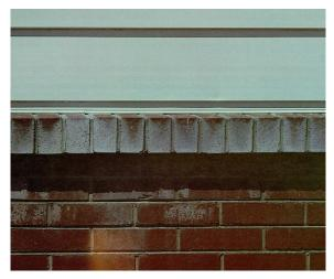
Chalking paint is deteriorated paint and must be repaired.
