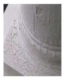
Cracking paint and cracked paint at a settlement crack is deteriorated paint and must be repaired when an adhesion test determines that any layer of paint is not securely bonded. To conduct an adhesion test, firmly press a 2" x 2" piece of masking tape to the suspect paint and rub the tape to adhere firmly. Lift up on one corner of the tape and remove the tape. If paint is evident on the tape, the paint is separating from the substrate or from underlying paint, and is not securely bonded.
