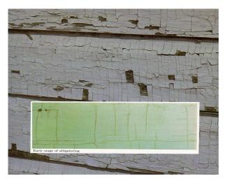
Alligatoring paint is deteriorated paint and must be repaired when an adhesion test determines that any layer is not securely bonded. To conduct an adhesion test, firmly press a 2" x 2" piece of masking tape to the suspect paint and rub the tape to adhere firmly. Lift up on one corner of the tape and remove the tape. If paint is evident on the tape, the paint is separating from the substrate or from underlying paint, and is not securely bonded.
