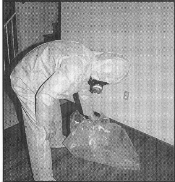
Figure 14.8b Fold Plastic Inward.
