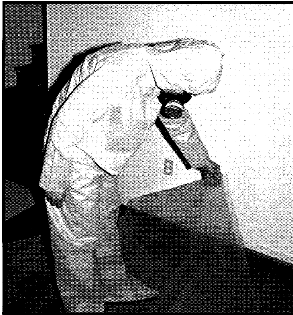
Figure 14.8a Pick Up Corners of Plastic Sheeting.
