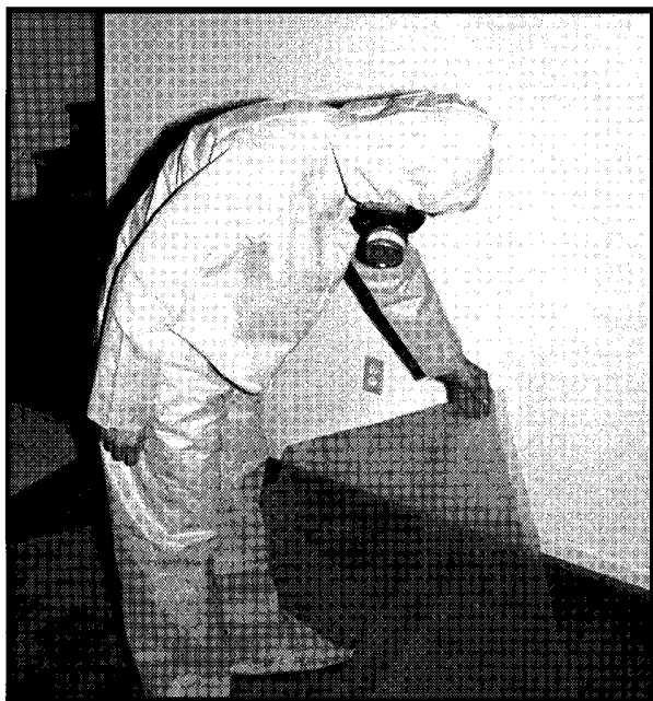
Figure 14.8a Pick Up Corners of Plastic Sheeting.
