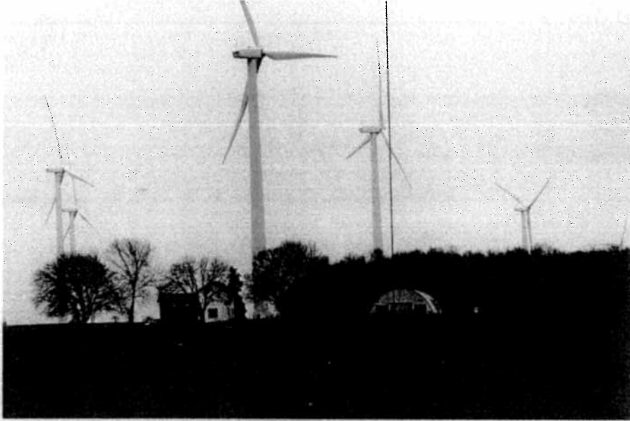
Fond du Lac County Home in PSC approved Wind Farm, April 2009
