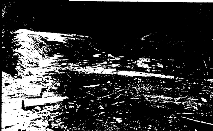
Figure 8 Highly acidic tailings, with high metals content, were released downstream following collapse of a tailings dam on the Rio Grande National Forest in Colorado.
