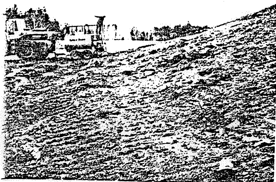
JCIC class 3 ore pile being hydroseeded in May 1981
