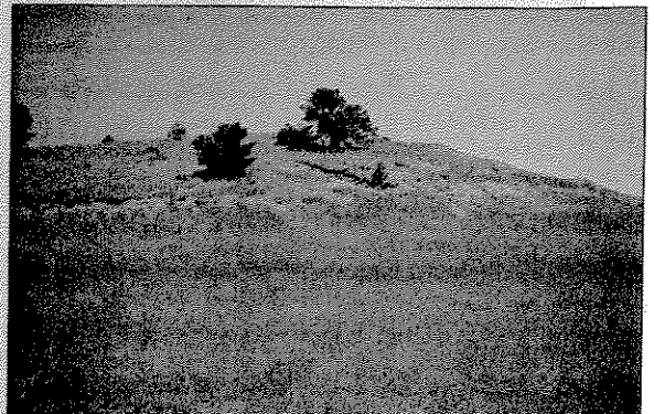
Right: Revegetation after two years. The line just beneath the trees is the uppermost diversion ditch separating reclaimed waste rock below from the natural slope and vegetation above.
