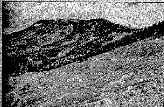
Right: Revegetation after two years. The line just beneath the trees is the uppermost diversion ditch separating reclaimed waste rock below from the natural slope and vegetation above.
