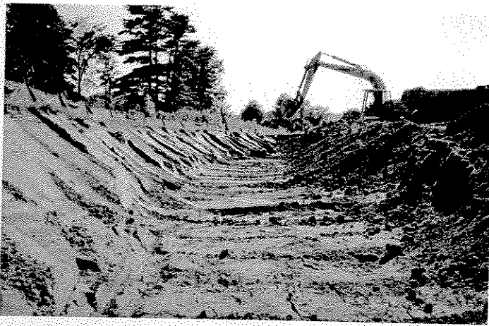
Wetland creation involves costly earth moving, making it a more expensive alternative than wetland restoration.
